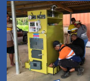
Assemble at the installation location
